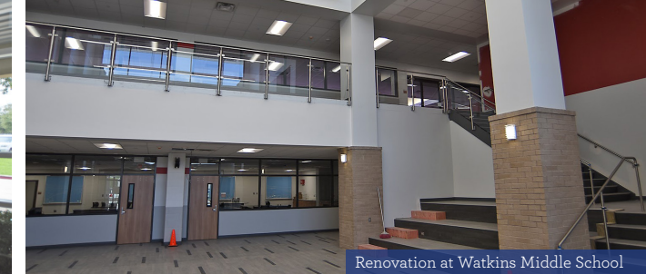
Renovation at Watkins Middle School
