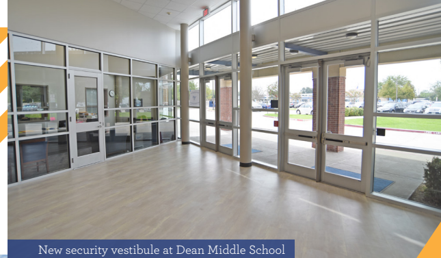
New security vestibule at Dean Middle School
