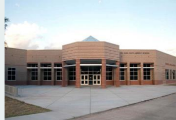
5. Bleyl Hub (data center)
